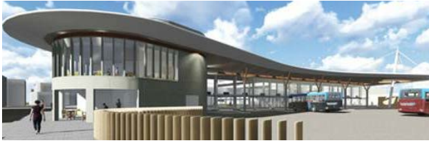
WALKING DISTANCE TO GLOUCESTER RAILWAY & BUS STATIONS
